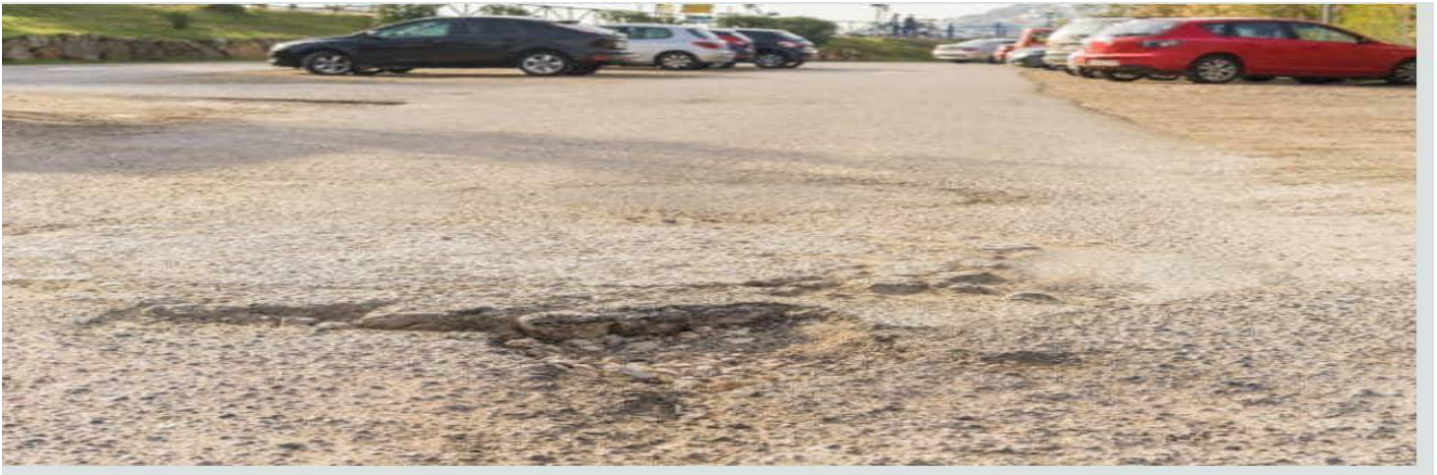
Plate 1: Pothole causing Traffic Obstruction along Felele Road, Lokoja
