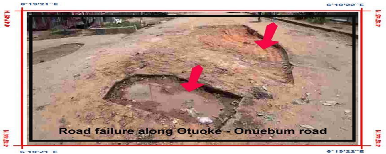
Figure 2: Image of failed portion of Otuoke – Onuebum road.
