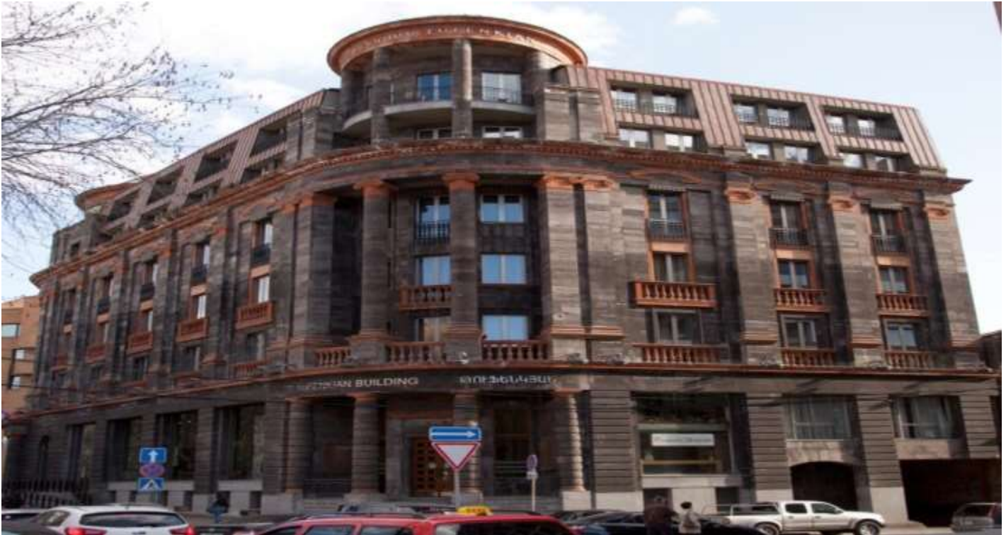
Figure 2. View of the 7-story base isolated “Tufenkian” building with non-symmetric plan of the multifunctional hotel/commercial center complex constructed in Yerevan
