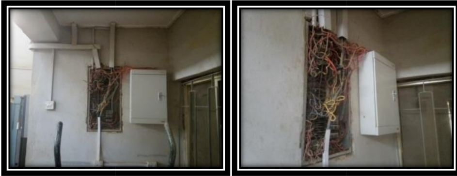
Figure 2A and B: A poorly executed electrical installation: untidy and aesthetically assaulting. It is a common feature in many Nigerian buildings or structures.
