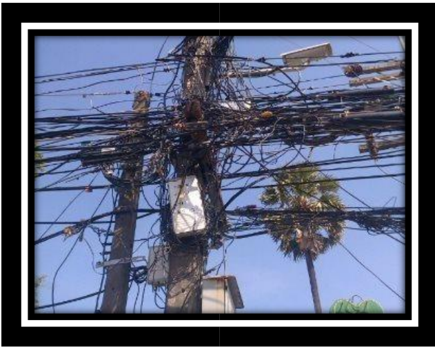
Figure 6: A functional but aesthetically poor and hazardous electrical installation. Source: Arrive Alive (2018).
