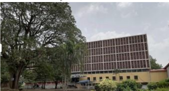
Figure 18: Use of Brise soleil as shading device of the Kenneth Dike Library University of Ibadan. Source: Researchers fieldwork
