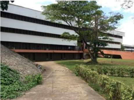
Figure 17: Use of horizontal concrete fins as shading device of the Hezekiah Oluwasanmi Library, Obafemi Awolowo University. Source: Researchers field work
